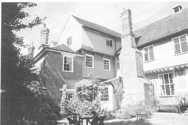
Fig 10: New 3-storey Stair Tower to left of chimney stack at Hadleigh Guildhall
