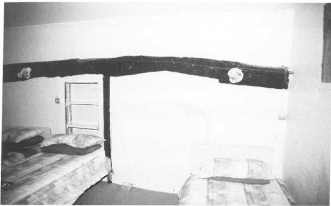
Fig 4: Fireplace in Service Chamber of Valley Farm
